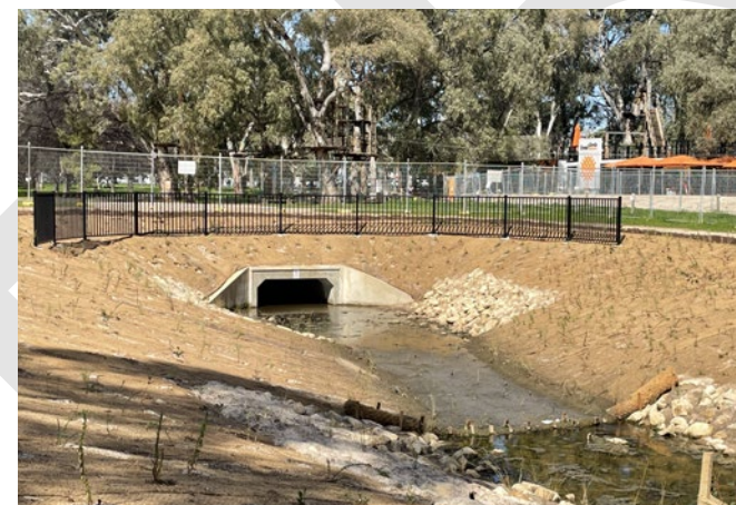
Park 20 new culvert and swale
