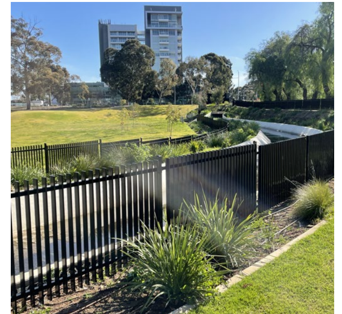
Concrete swale and fencing
