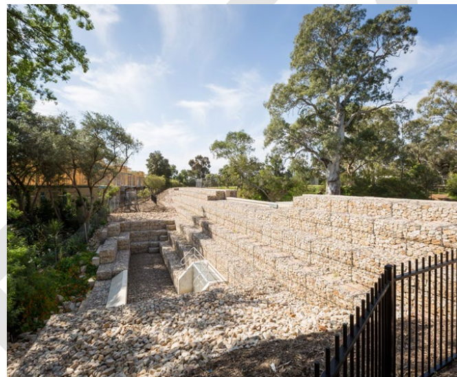
Flood Control Dam
